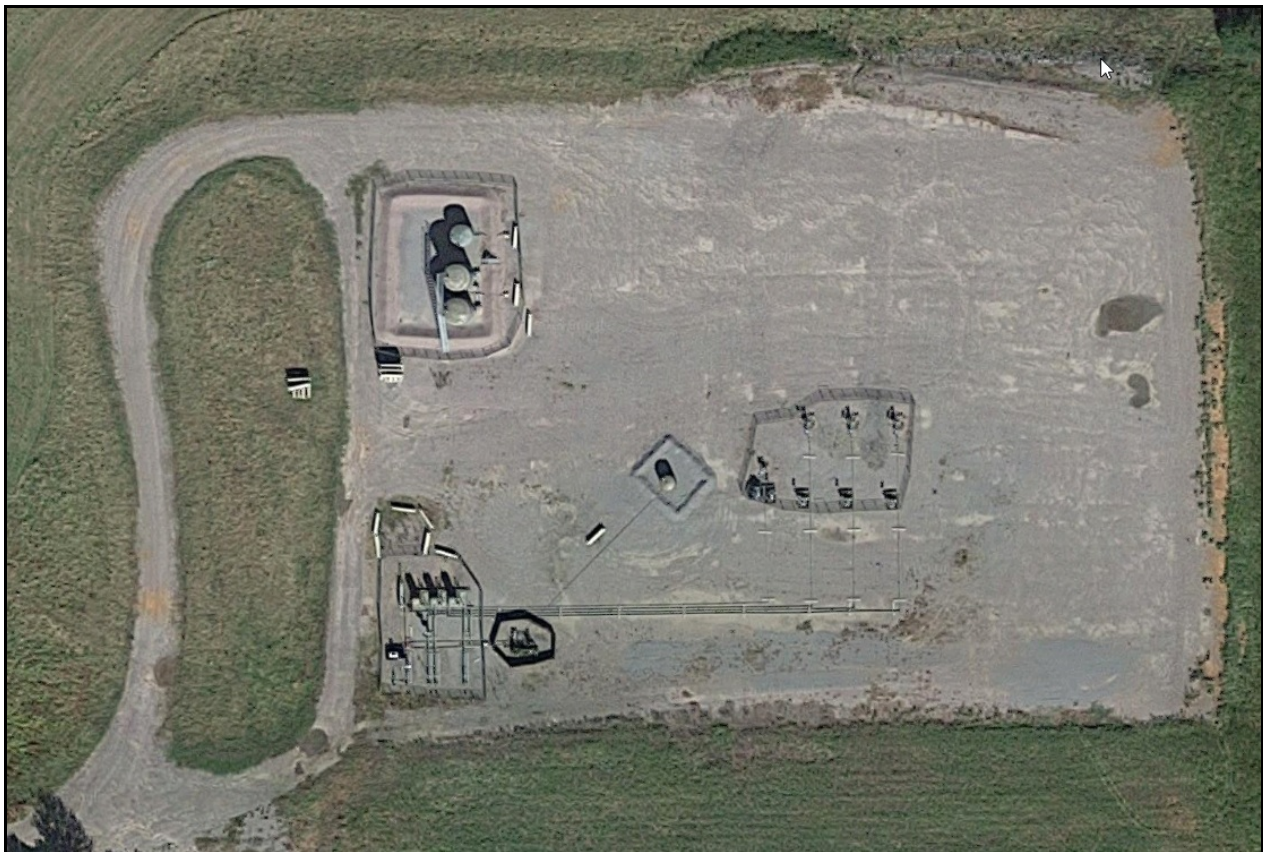
Exhibit 6.1-1: Typical Fayetteville Shale Gas Pad
